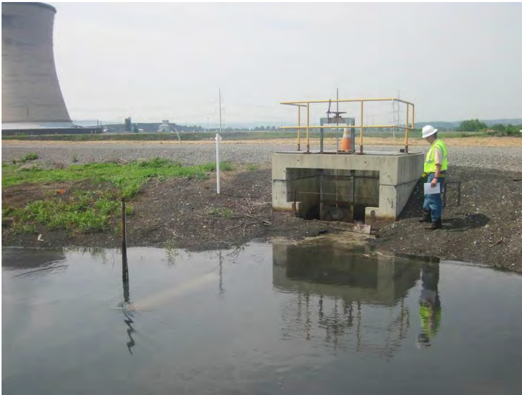
Photo 37 – Intake structure at the splitter dike.
