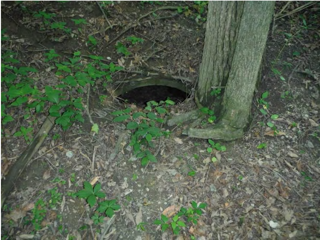
Photo 41 – The outlet pipe of an abandoned outlet structure running from Sub-basin C to Chillisquaque Creek.
