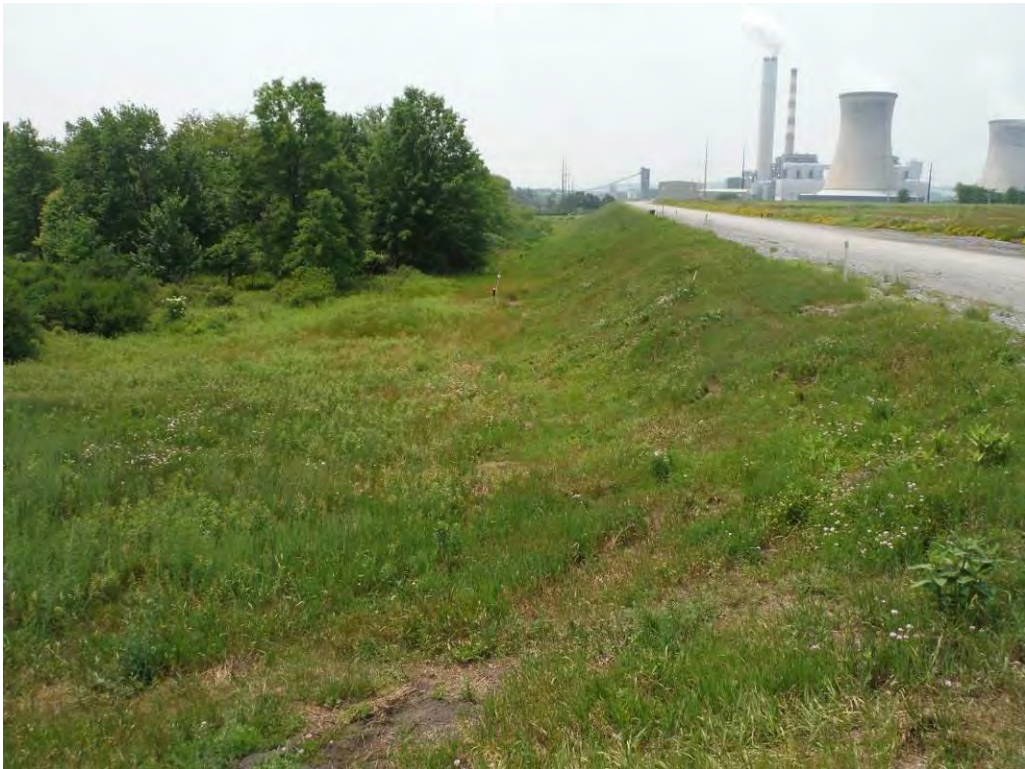
Photo 22 – The south downstream slope of Sub-basin A, looking west.
