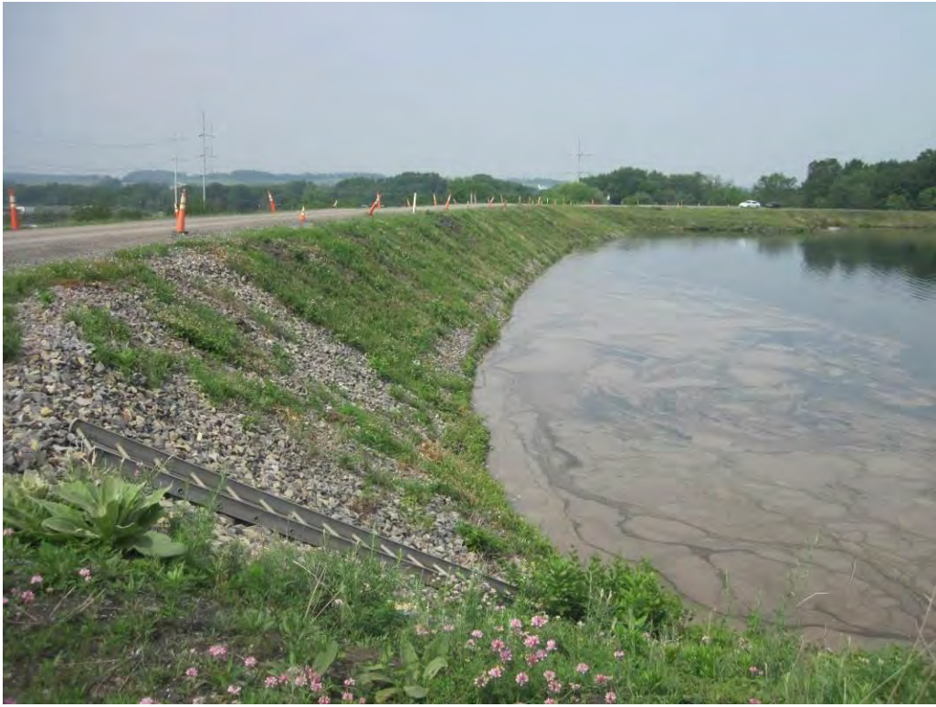
Photo 5 – Upstream slope of Sub-basin C looking northwest, showing riprap slope stabilization.
