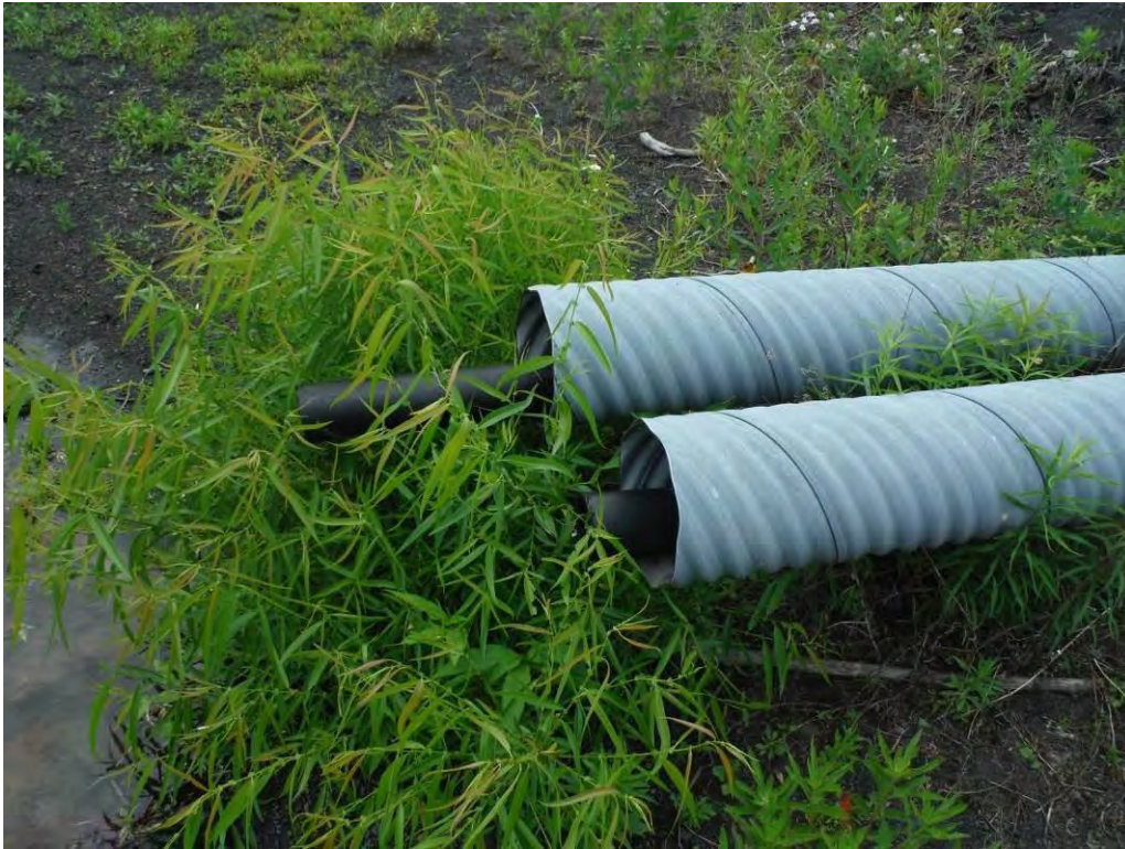
Photo 9 - Middle dewatering well discharge area. No significant deposition was observed.
