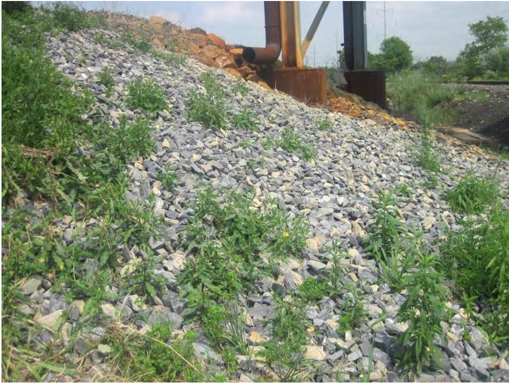
Photo 31 - Riprapped slope at the footing for the pipe bridge.
