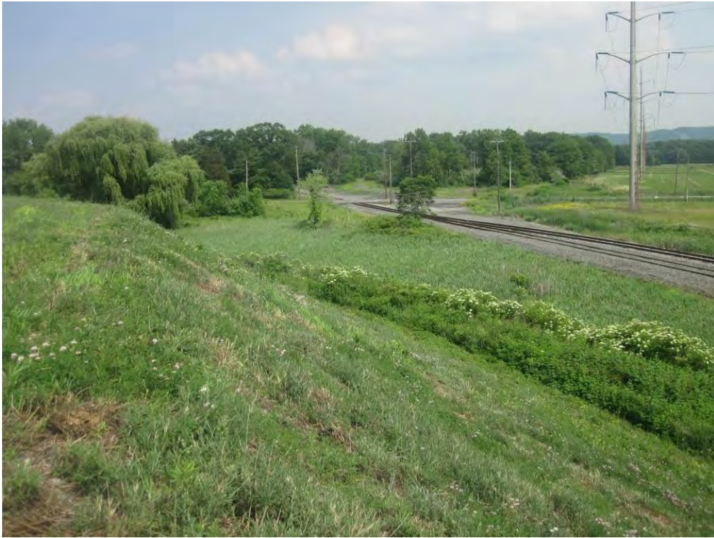
Photo 21 – Southwest corner of the basin, looking southeast. A depression noted in previous reports at southwest corner of the basin, measuring 5 feet wide by 3 feet deep, was not visible due to overgrown vegetation.
