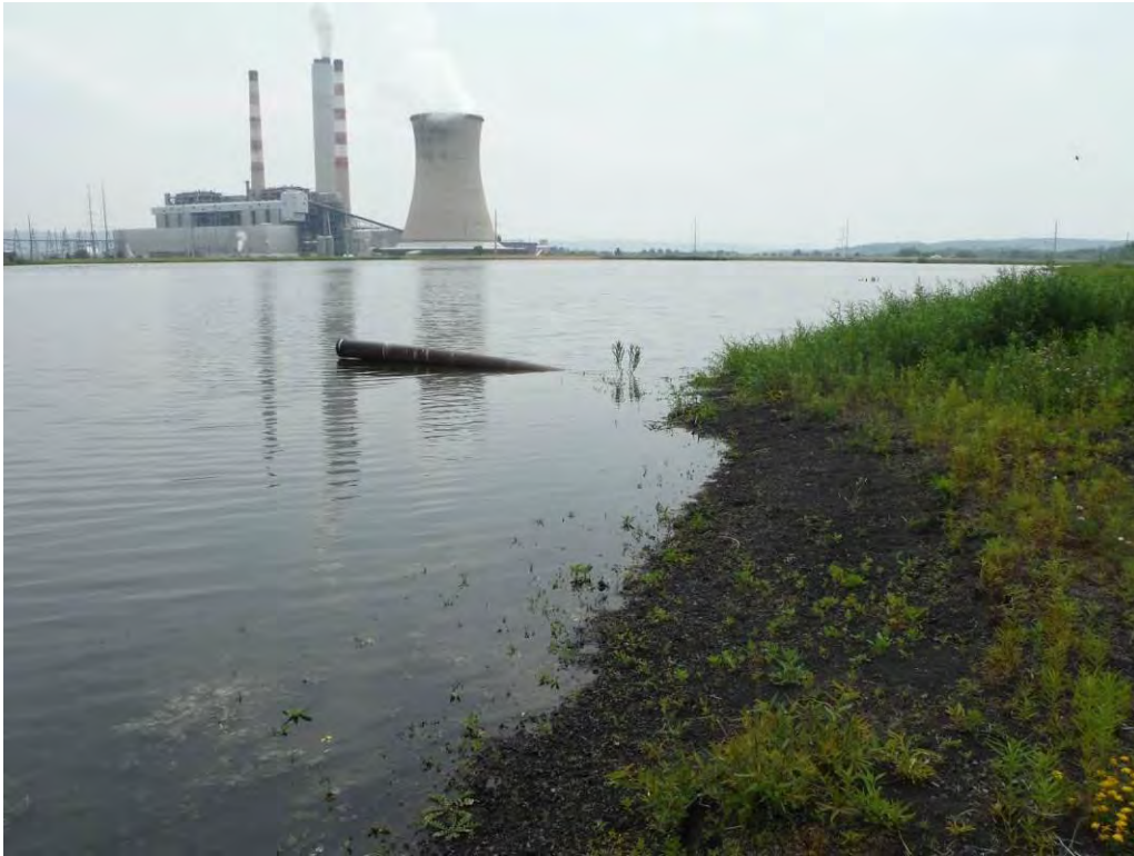
Photo 7 – Upstream slope of Sub-basin B showing the 12-inch HDPE extending into the basin in the background. This pipe is believed to be a discontinued ash deposition line, and the orientation and means of closure of the buried part are not known.
