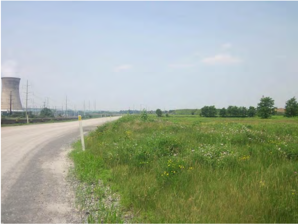
Photo 11 – Closed area of Sub-basin A, adjacent to the southwest embankment.
