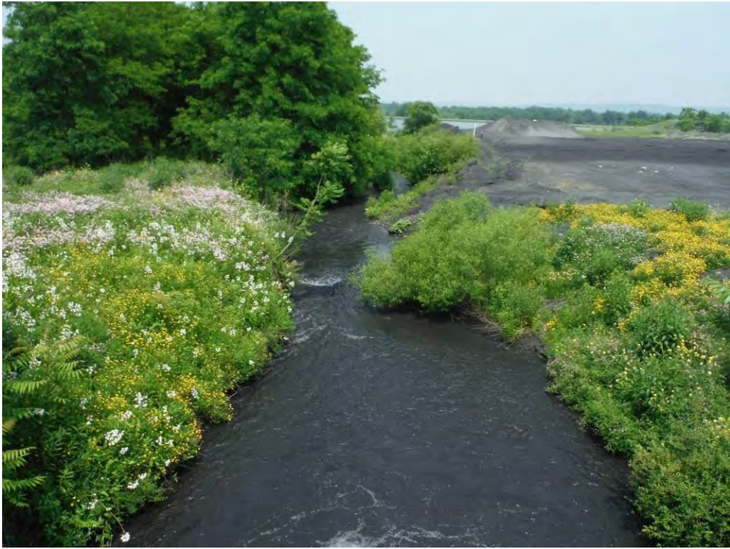
Photo 35 – Discharge channel from the ash slicing area to Sub-basin B. Note the narrow channel and steep side slopes.
