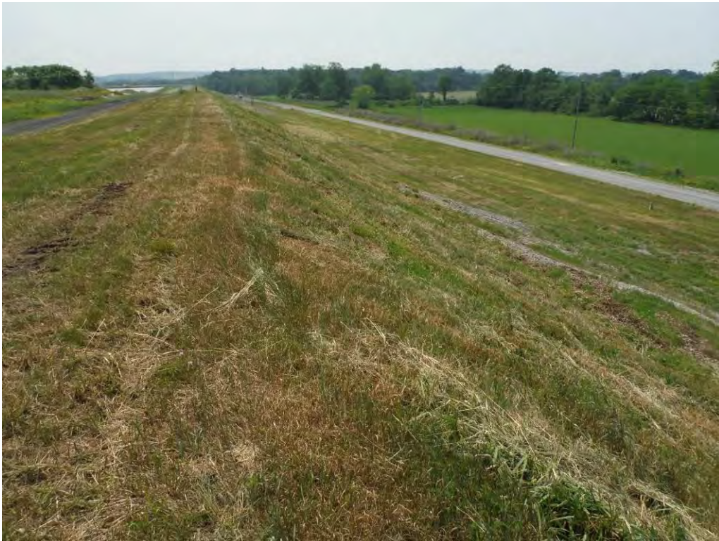
Photo 26 – Looking west along the downstream slope of the north embankment.
