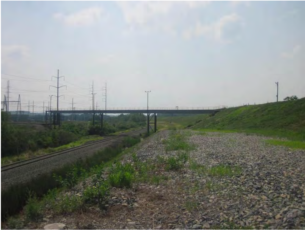
Photo 19 – Crest of stabilization berm along the southwest embankment, looking northwest from southwest end.
