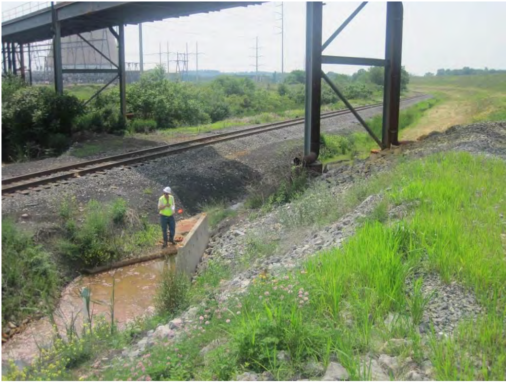
Photo 32- Slope stabilization at embankment toe near pipe bridge footing.
