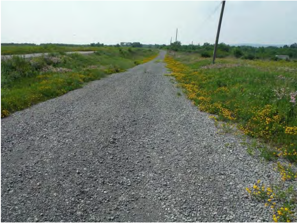
Photo 23 – Crest and downstream slope of Sub-basin A, looking north.
