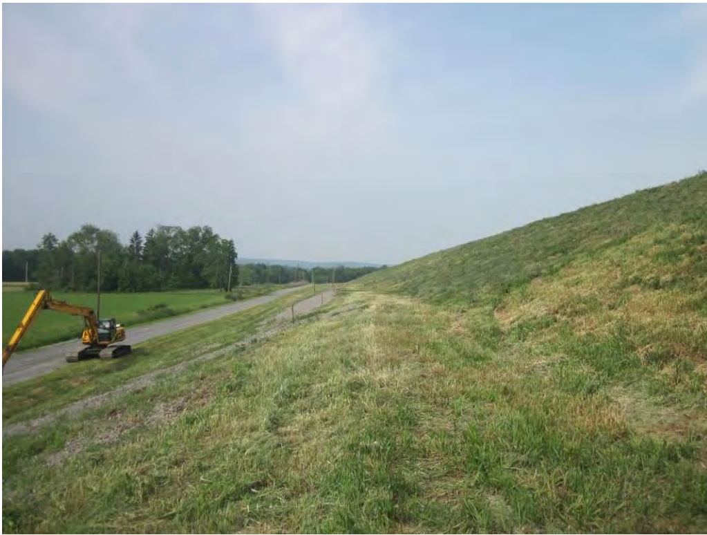
Photo 27 – The downstream slope of the north embankment, looking east.
