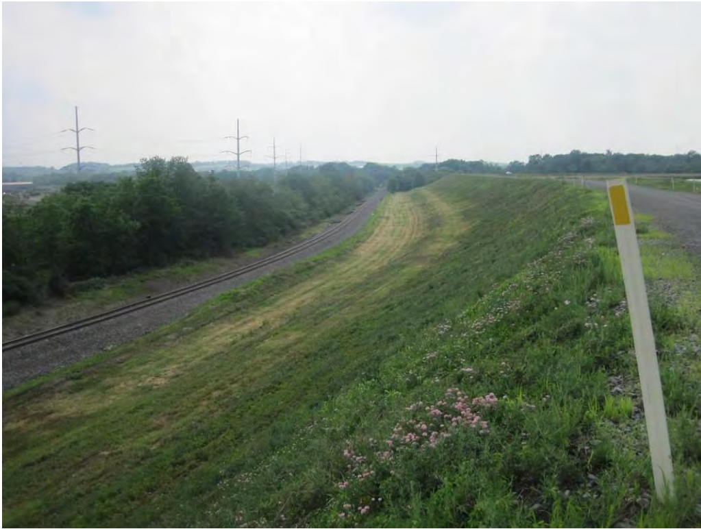
Photo 17 – Downstream slope of the southwest embankment, looking northwest from pipe bridge. Standing water had been observed previously along the stabilization berm where the tracks are, although this area was comparatively dry in 2015.
