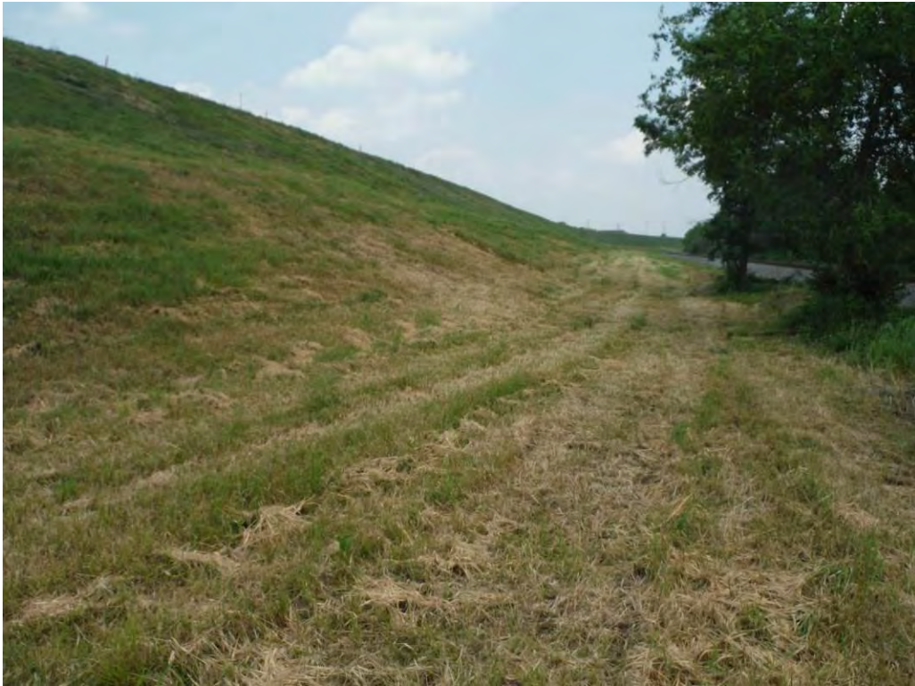
Photo 15 - Stabilization berm along the northwest end of the southwest embankment.
