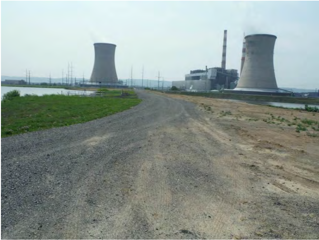
Photo 6 – Splitter dike between Sub-basin B and C, showing the vegetated bottom ash bench against the inside slope of Sub-basin B, effectively widening the embankment.
