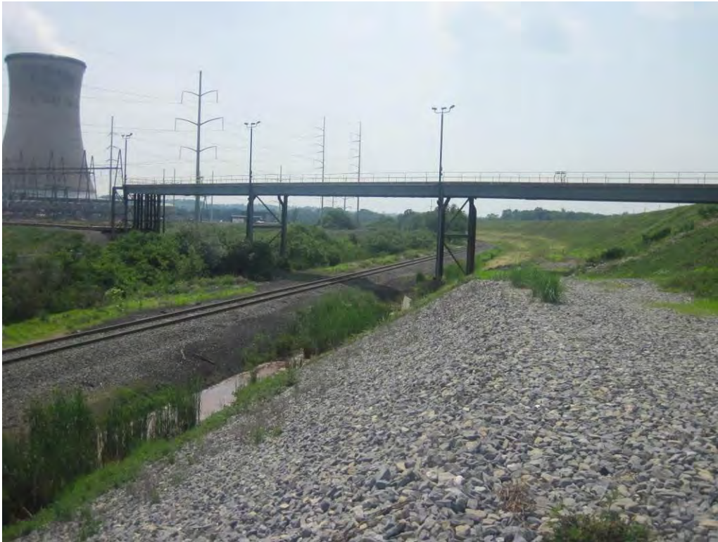
Photo 30 – Pipe bridge crossing the southwest embankment.
