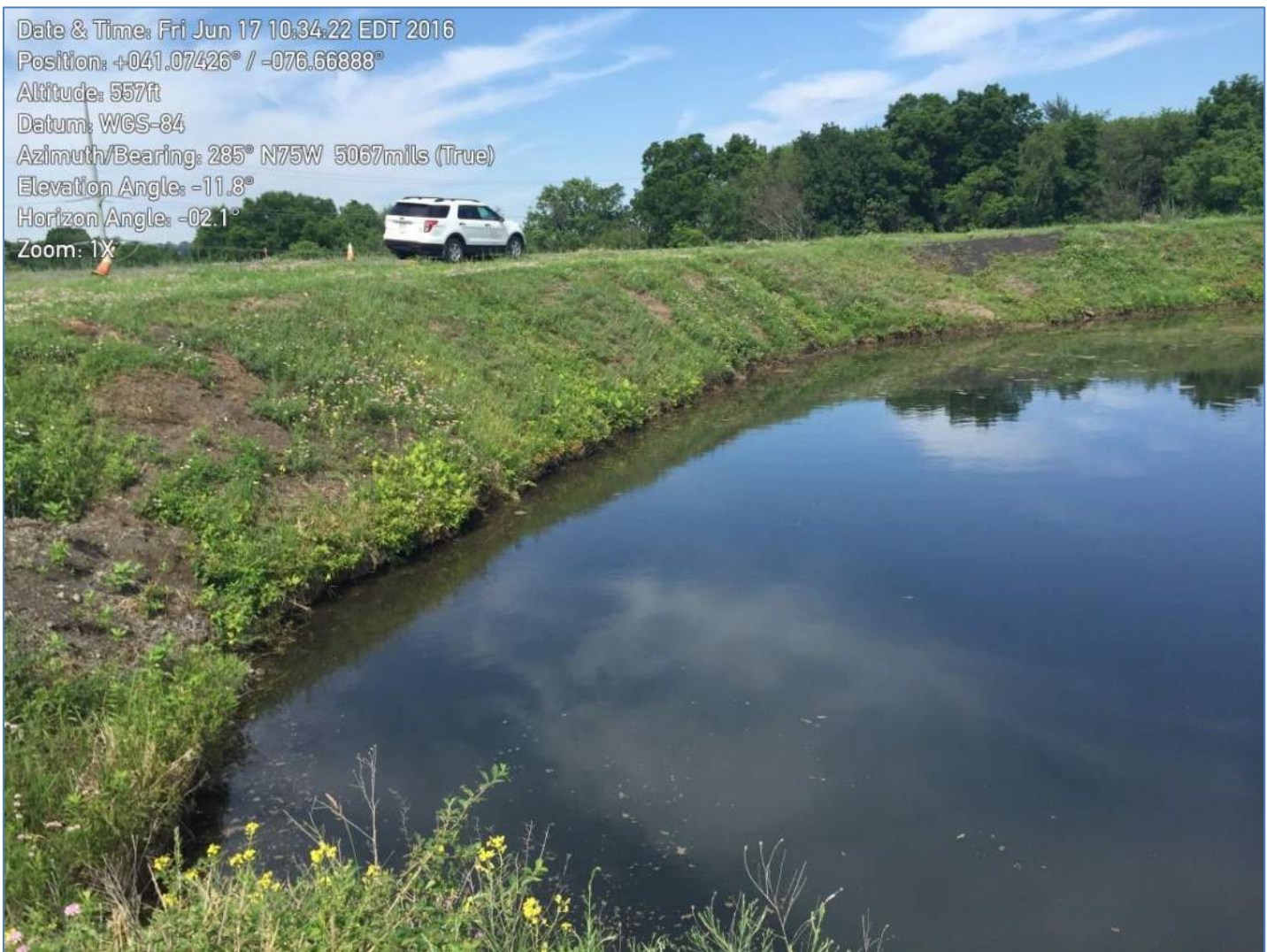
Photograph 5 – Western Upstream Slope of Subbasin C
