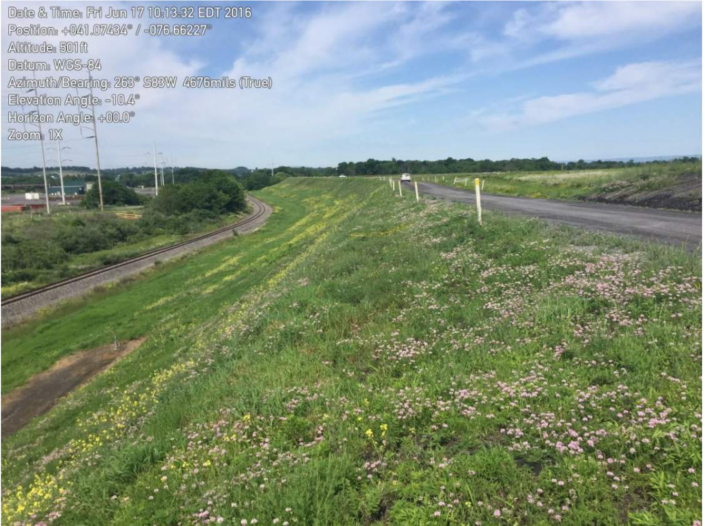
Photograph 13 – Southern Downstream Slope and Dike Crest (looking west)
