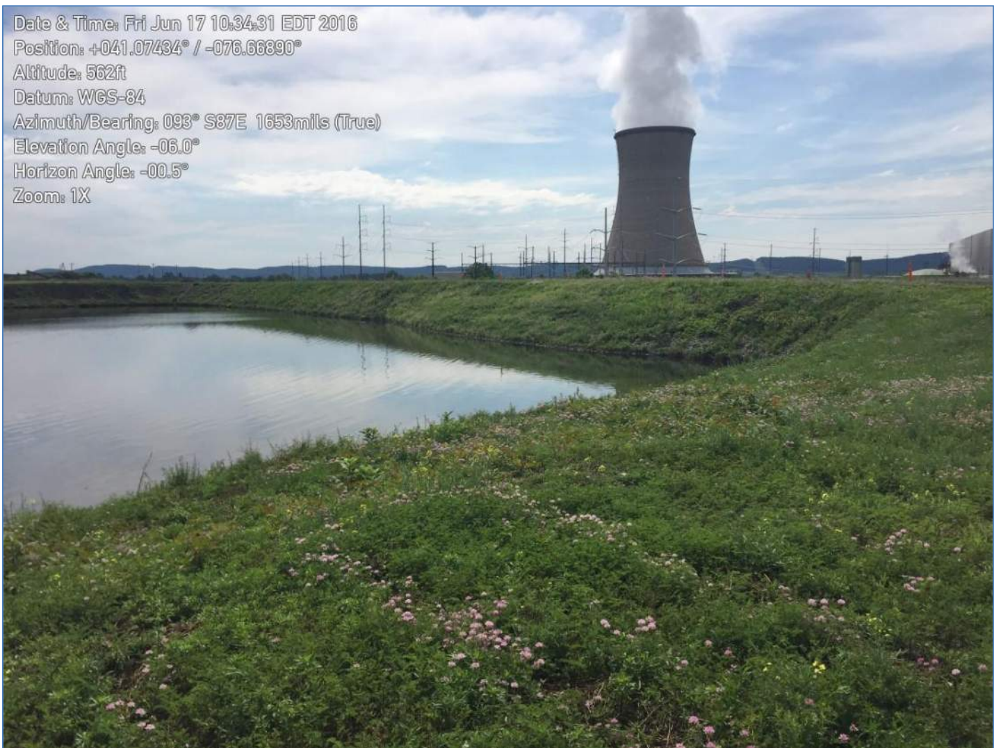
Photograph 6 – Southern Upstream Slope of Subbasin C
