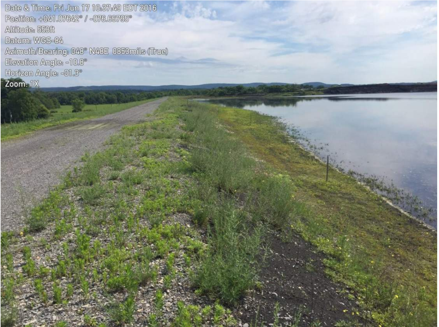
Photograph 7 – Northwestern Upstream Slope of Subbasin B (looking northeast)
