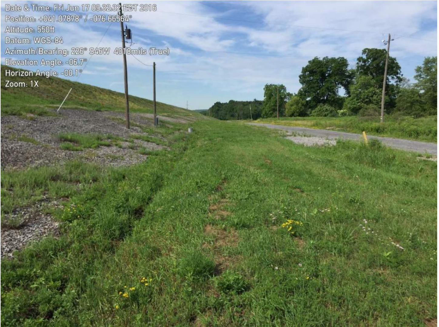
Photograph 11 – Northern Downstream Slope (looking west)
