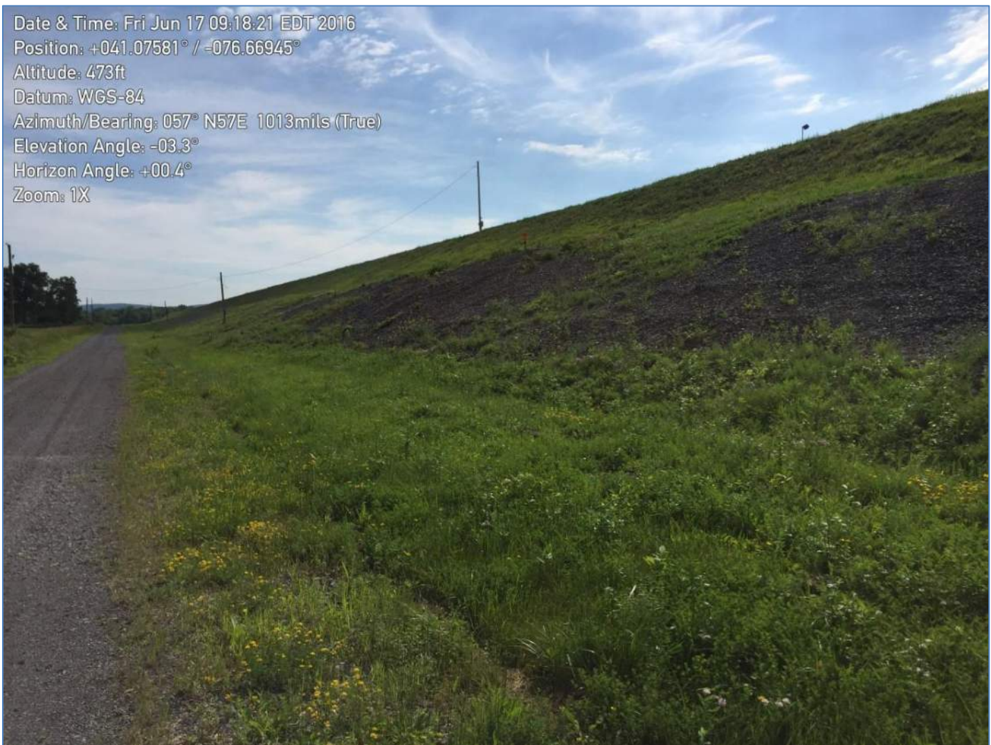
Photograph 12 – Northern Downstream Slope (looking east)
