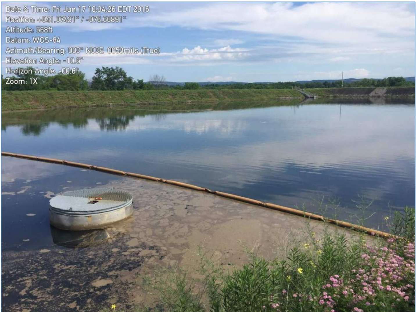
Photograph 8 – Top of Spillway Riser in Subbasin C (looking north)
